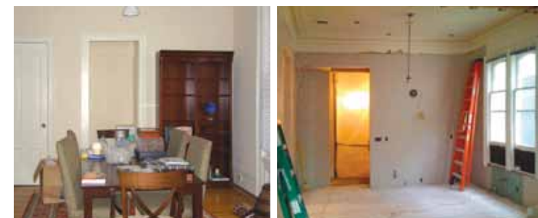
The kitchen moves into the parlor. The original house had a pair of parlor rooms separated by tall pocket doors. The street-side parlor was a sitting room, the other a dining room (photo above left). In the revamped space, the pocket doors have been removed, the hall is redirected to enter the kitchen (photo left), and the lower sashes of the double-hung windows are shortened (photo above right).
